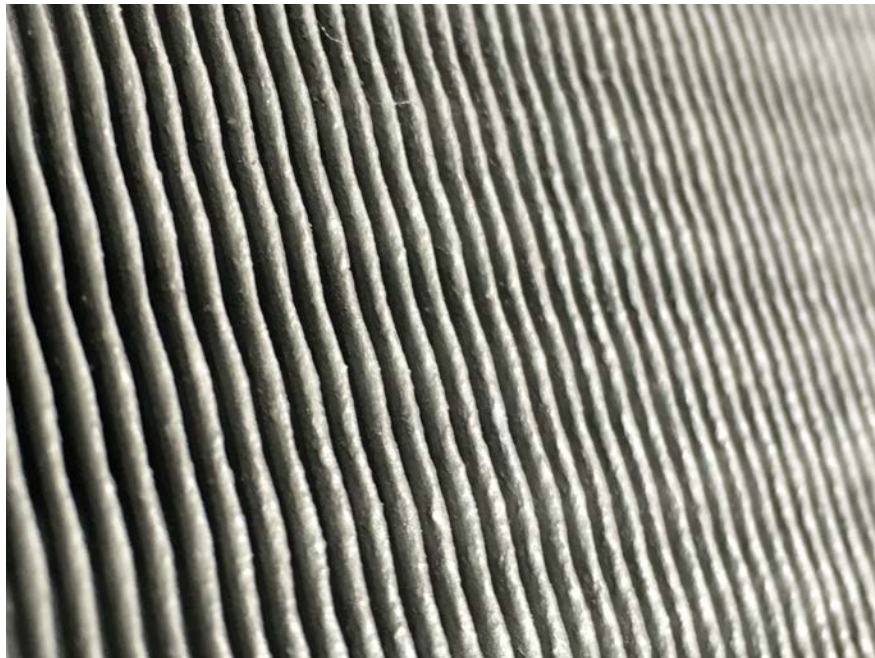
Figure 30 ACU-14, 160 tons, Condenser Face, Treated Close-up
