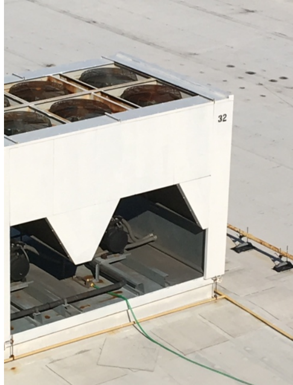
Figure 16 Mammoth ACU-32, 110 tons
