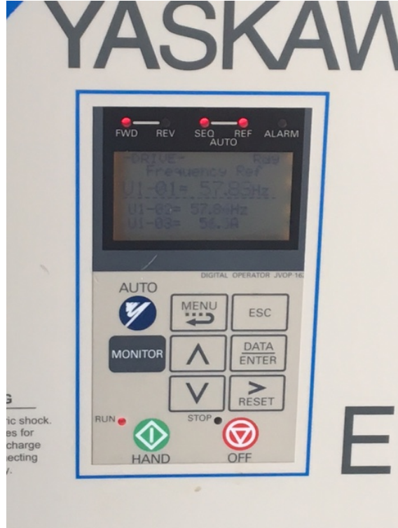
Figure 10 Mammoth ACU-34 VFD, 57.89 Hz, 96.5% speed
