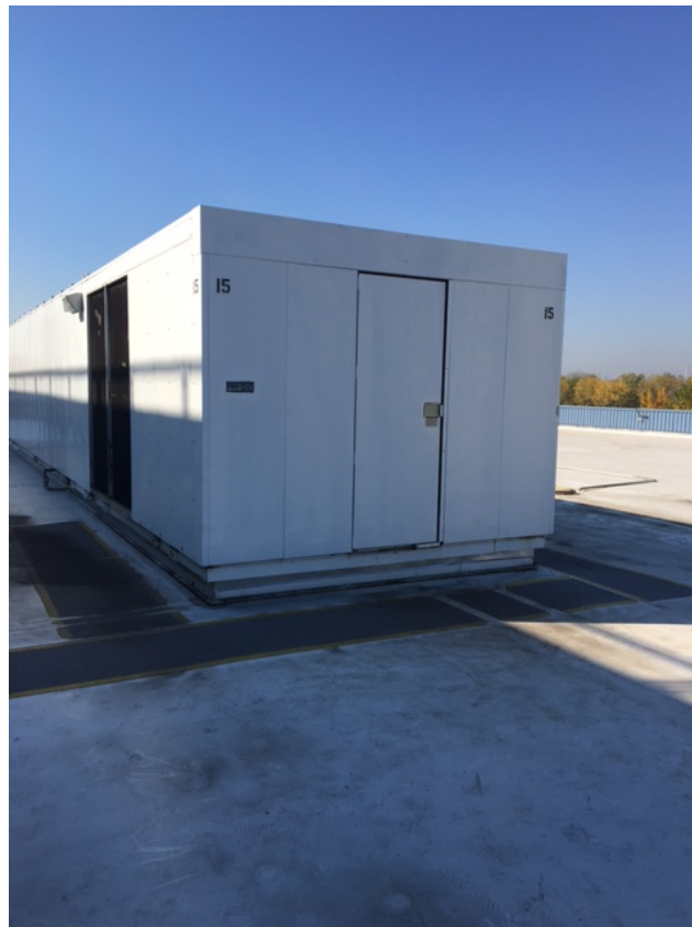
Figure 17 Mammoth ACU-15, 160 tons
