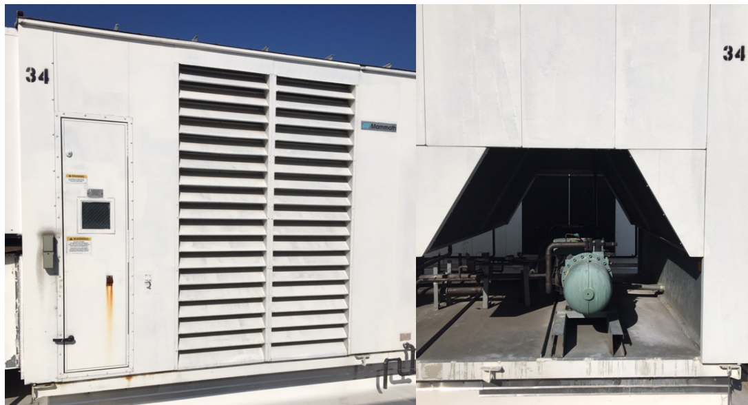
Figure 9 Mammoth ACU-34, 170 tons
