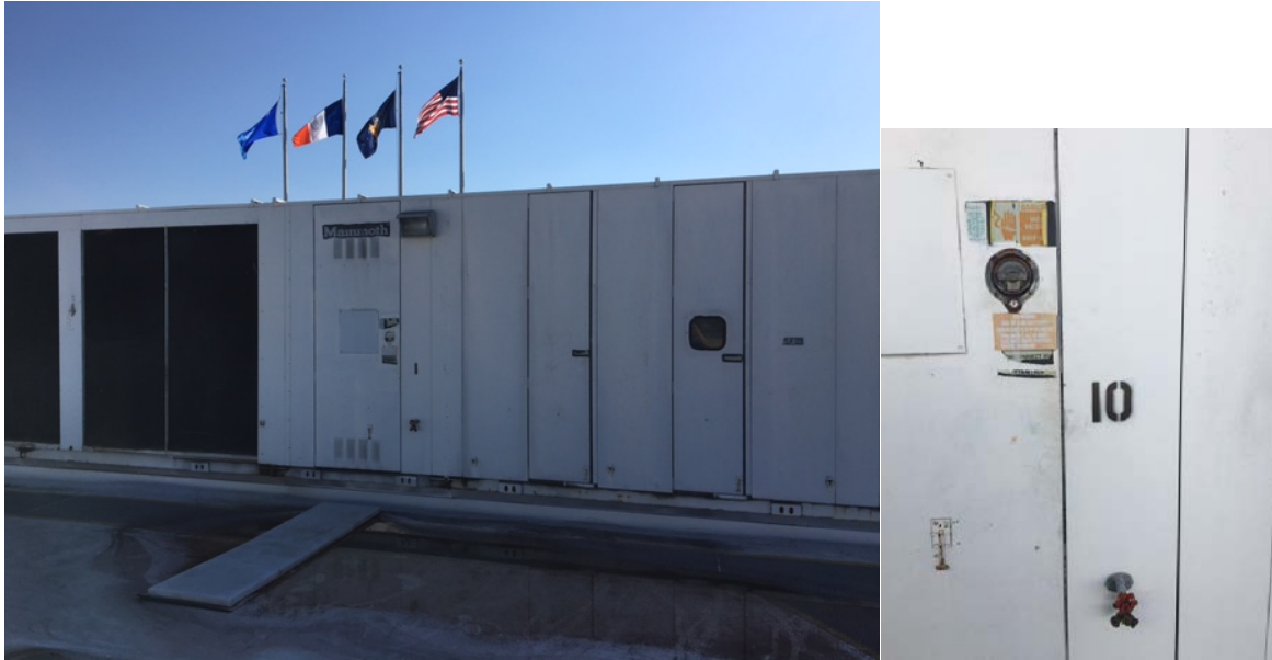
Figure 6 Mammoth ACU-10, 150 tons
