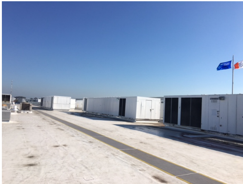
Figure 3 Mammoth ACU 2, 7, & 9 - 150 tons each
